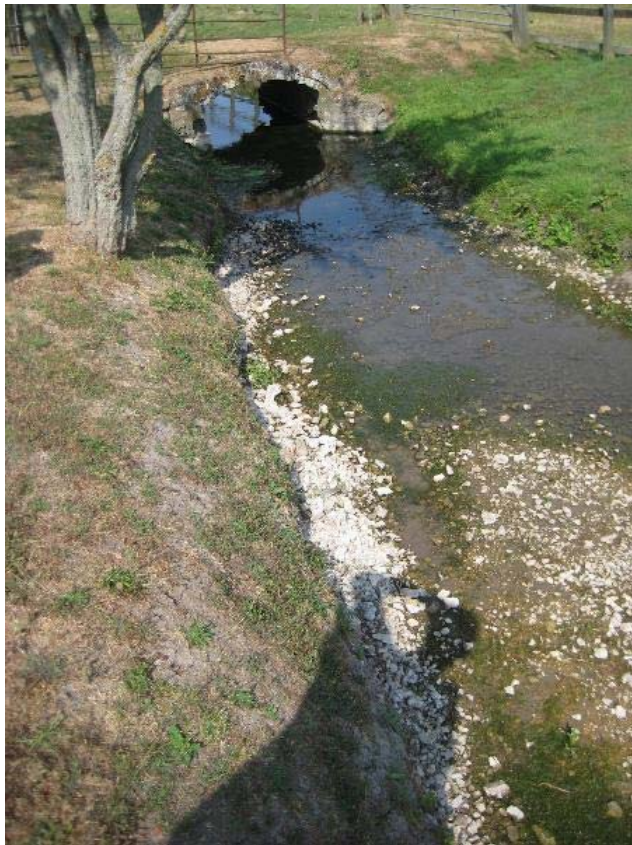
Photograph 8.6.5: Footbridge with a side bar starting to mature in the foreground. Caker Stream (facing downstream), 24/07/18, standard lens
