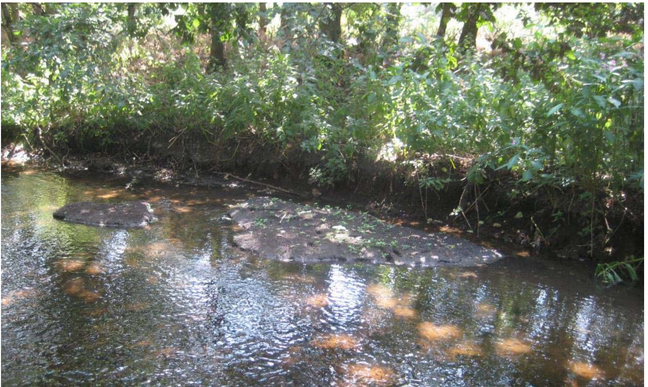
Photograph 8.6.22: Depositional feature showing signs of vegetation. Left bank is showing signs of undercutting. River Blackwater (right bank to left bank), 25/07/18, standard lens.
